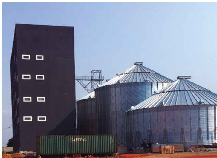
External view of the Ocrim plant for the Sanabel Group.
